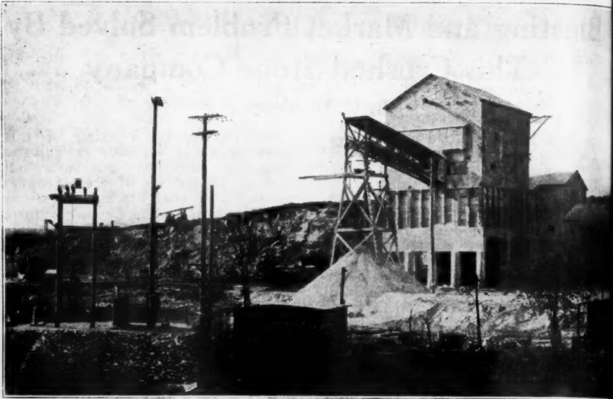
The Layout of the Plant is Particularly Ad
